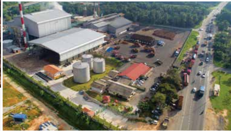
A 7MW biomass plant at Tenaga Sulpom Sdn. Bhd., Dengkil, Selangor.
