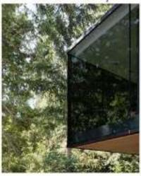
Full switching under 3 minutes provides energy efficiency and near-privacy. Visible transitioning within 20 seconds
