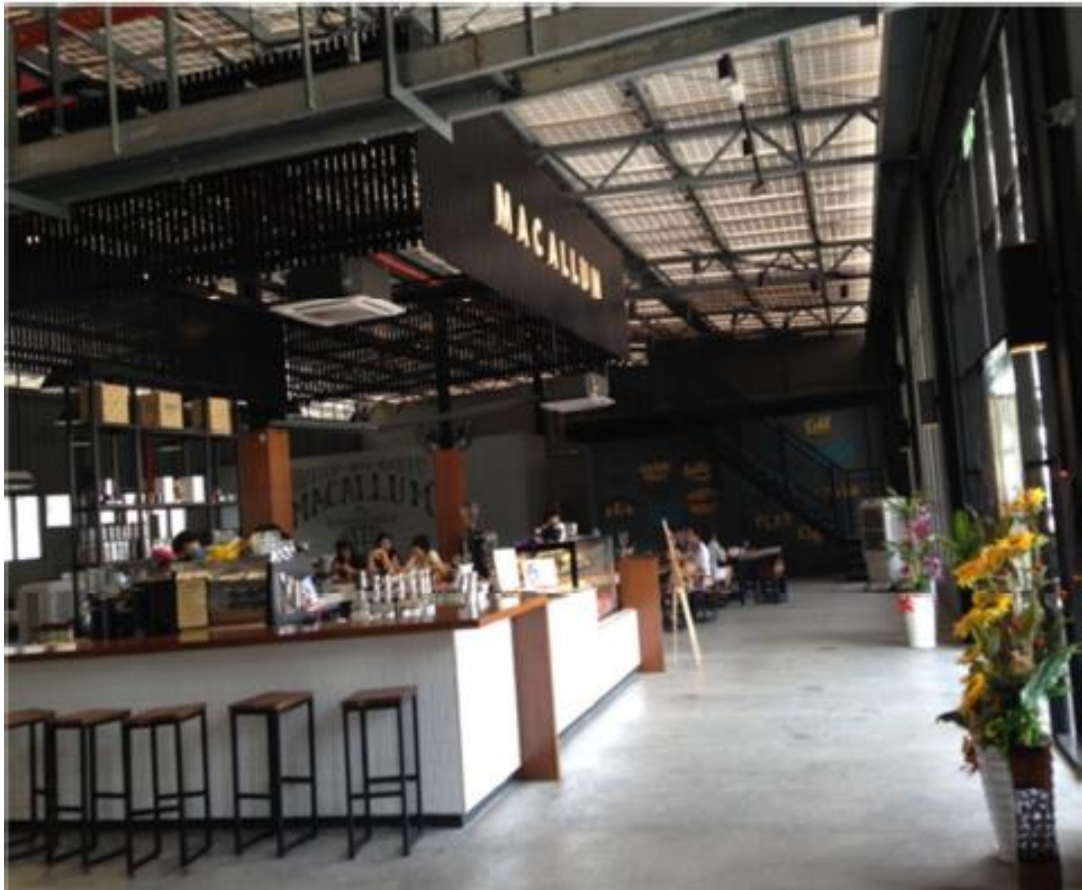
Figure 26 - Restaurant With PV Modules As Roof
