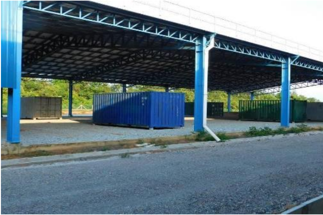
Figure 34 - The Area Below The Building Is Not Fully Utilized. Cabins Need Not Be Stored Under Shade
