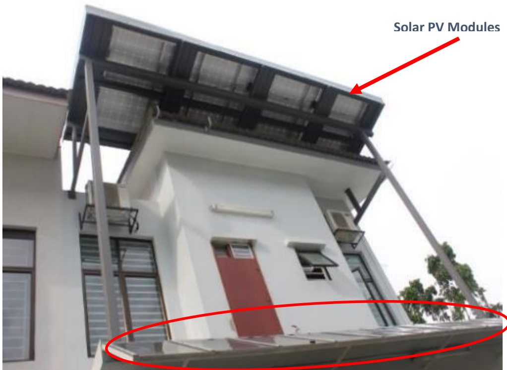
Figure 4 - A Secondary Roof Beneath The Modules Serving The Same Function
