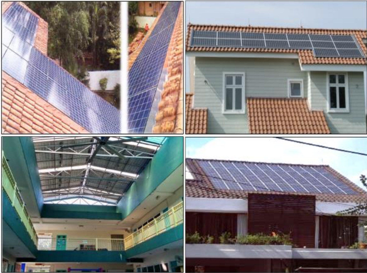
Figure 1 – Solar PV: Use as Roofing Material
