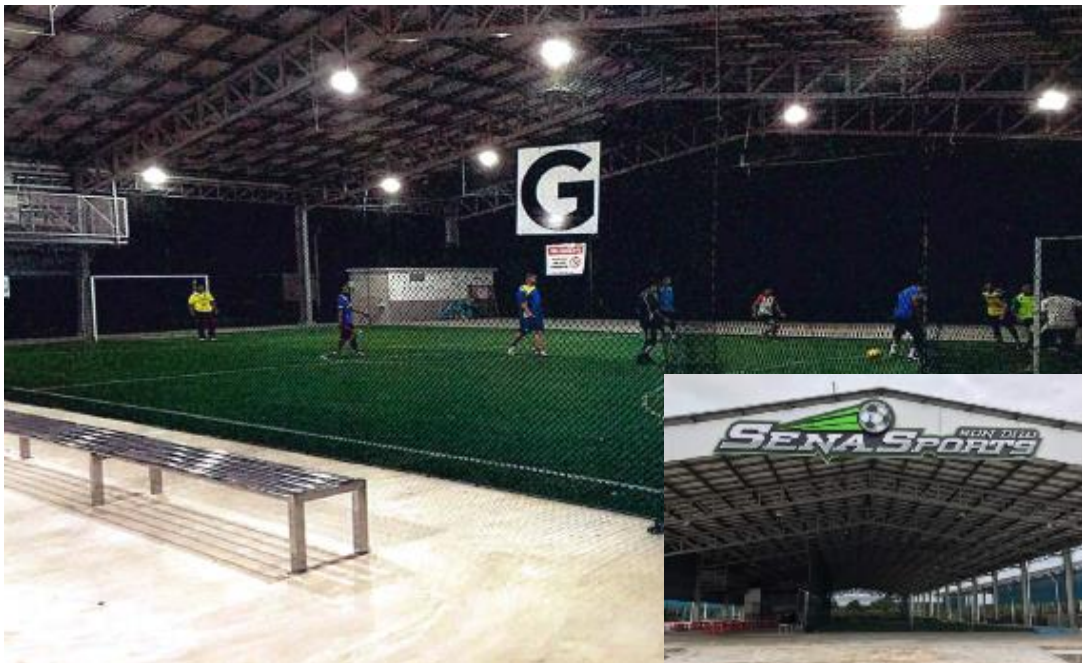
Figure 27 – Futsal Court with PV Modules as Roof
