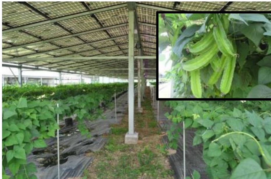
Figure 18 - Agriculture Produce (Four Angled Beans) Growing Healthily – subject to PV structure design which allow sufficient amount of sunlight for the crops
