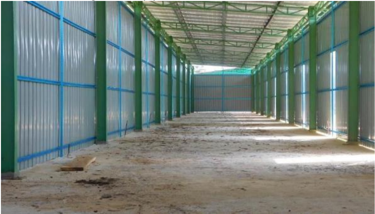
Figure 31 - Warehouse Which Serves No Function
