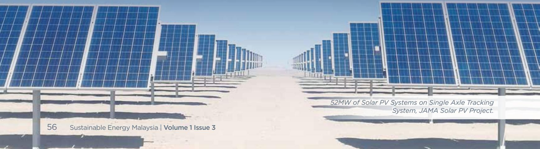
52MW of Solar PV Systems on Single Axle Tracking System, JAMA Solar PV Project.
