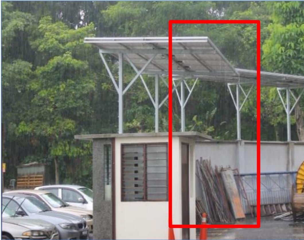
**Figure 17 - Installation serves no function or purpose(Walls Do Not Need Roof)**
