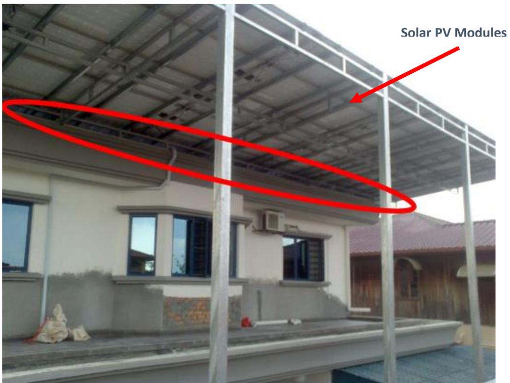
Figure 5 – Example 1: Overlapping Of Modules On Top Of Existing Roof
