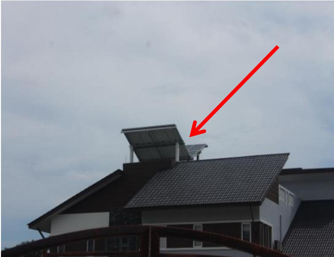
**Figure 10 - Installation Does Not Serve As A Primary Roofing Function**
