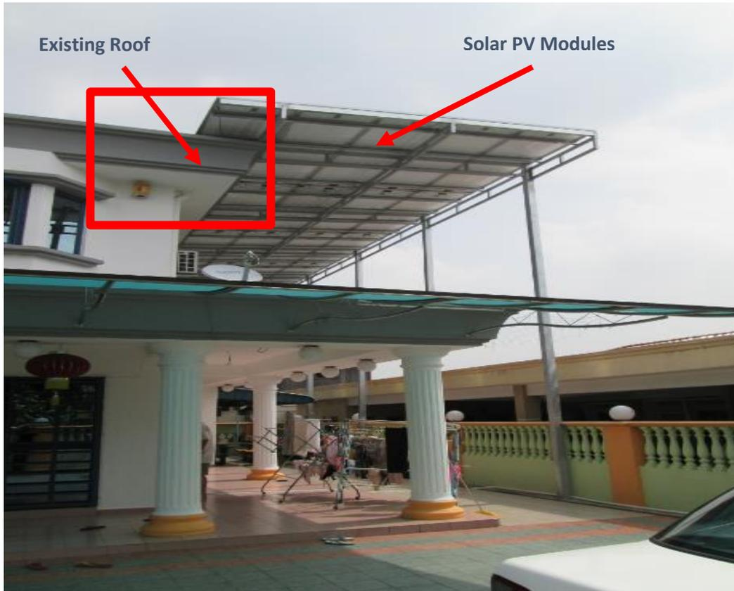
**Figure 6 – Example 2: Overlapping Of Modules On Top Of Existing Roof**
