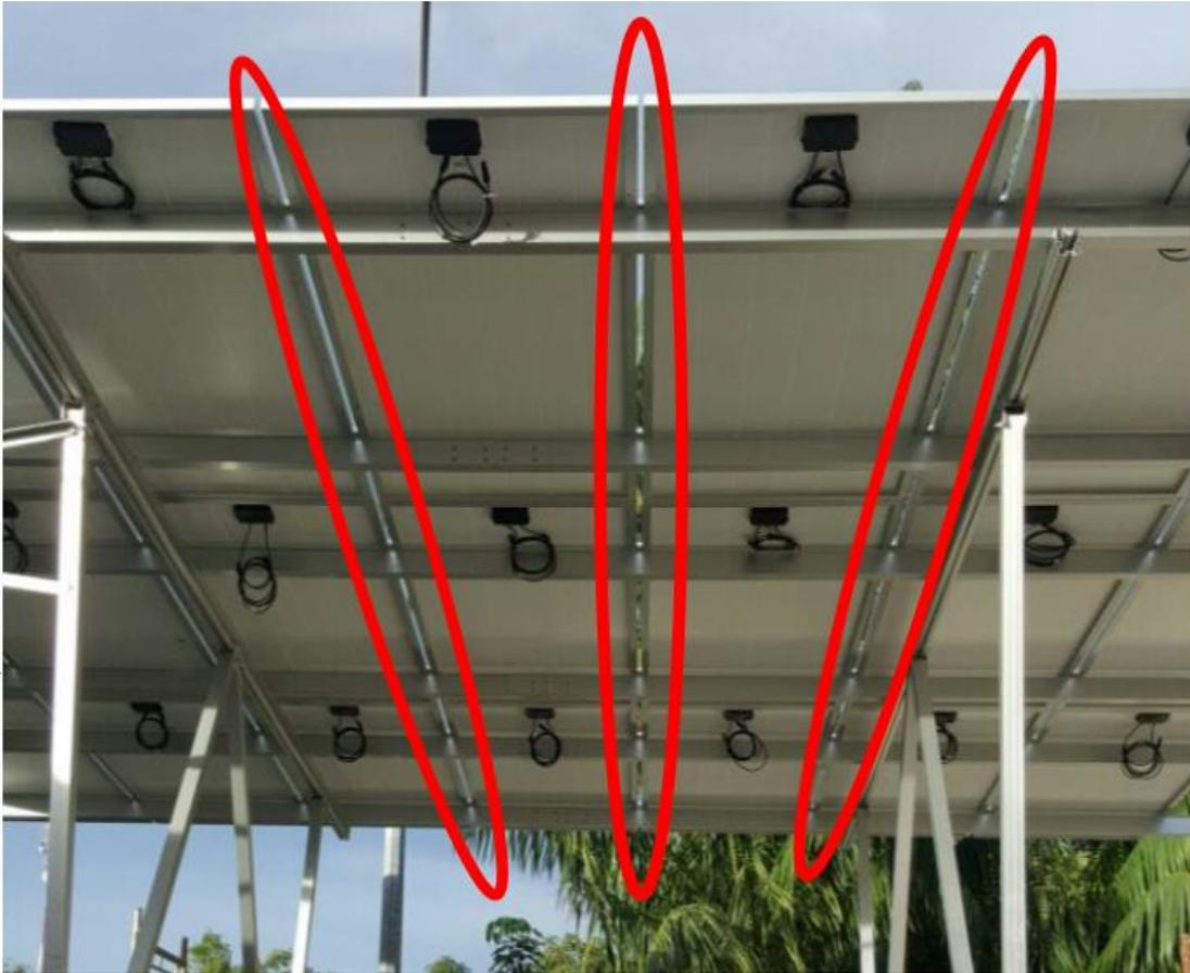
Figure 13 - Gaps Between PV Modules Are NOT Allowed
