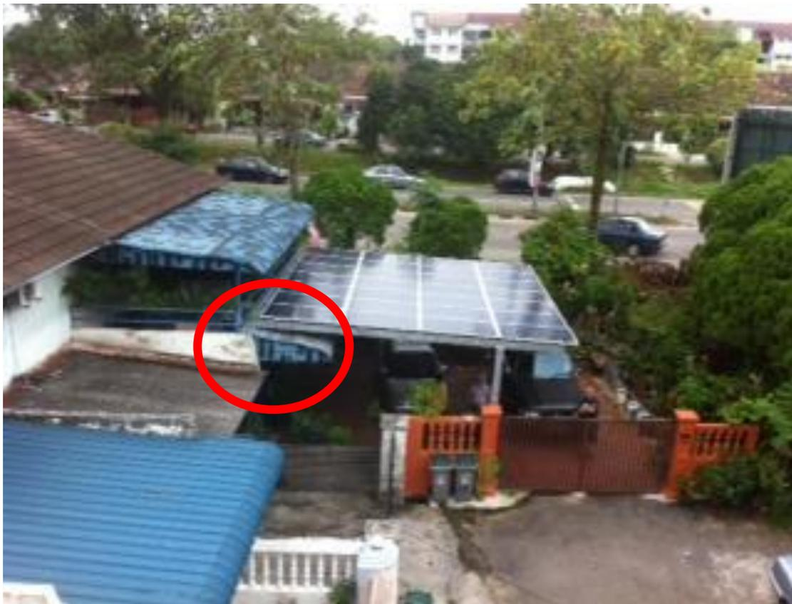
**Figure 7 – Example 3: Overlapping Of Modules On Top Of Existing Roof**
