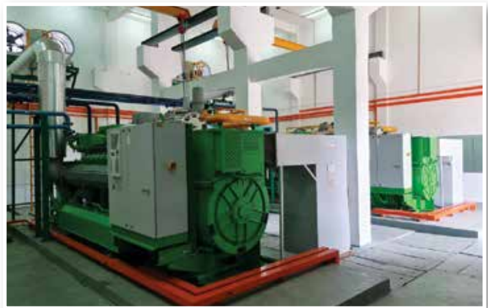
FGV's Triang biogas engine
