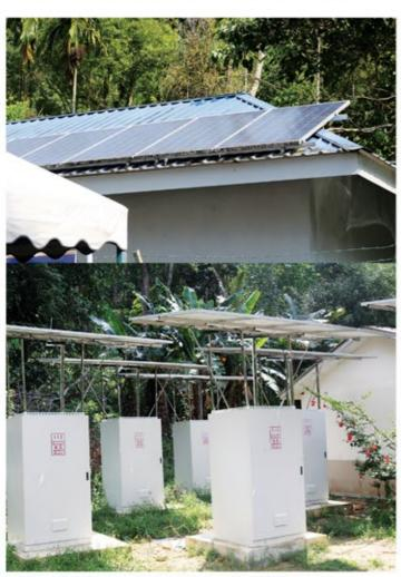
12 Orang Asal houses were equipped with 1.2kWp solar PV system including battery storage and basic electrical appliances such lighting and fan for every household
