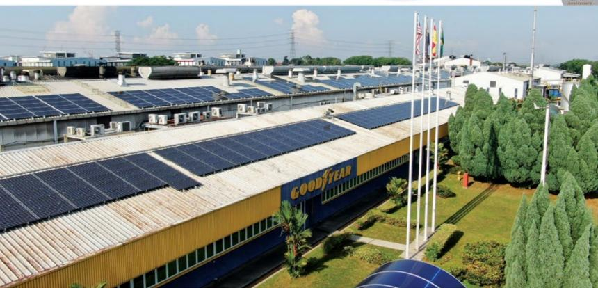
The 2.5MWp rooftop solar PV system installed at Goodyear Malaysia Bhd, Malaysia's project under NEM programme.
