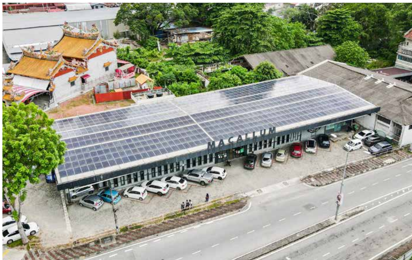
Pemasangan BIPV Solar 175.5 kW di Georgetown, Pulau Pinang. The 175.5 kW of BIPV Solar installation in Georgetown, Pulau Pinang.
