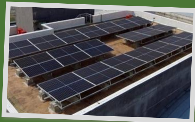
Sistem Solar PV 16kW di atas bumbung Galeria PJH di pejabat Pihak Berkuasa. The 16kW Solar PV system on the rooftop of Galeria PJH at the Authority's office.
